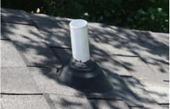
It seems that the rubber boots tend to deteriorate in approximately 5 years which leaves a hole in your roof. My lead stacks are not safe because squirrels like to sharpen their teeth on the lead.
